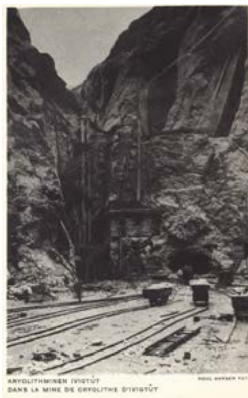
Figure 11. Picture postcard of the cryolite mine entrance at Ivigtût. Note the cryolite ore-cars on tracks (circa 1930).
