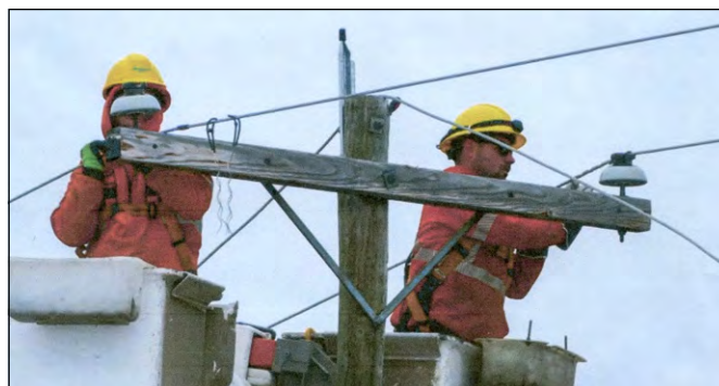
Figure 9. Working at installing new Hydro lines.
