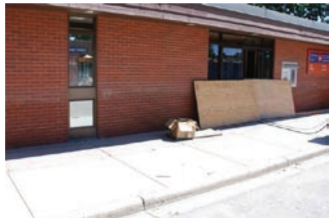
Figure 10 - close-up of flooded main post office.
