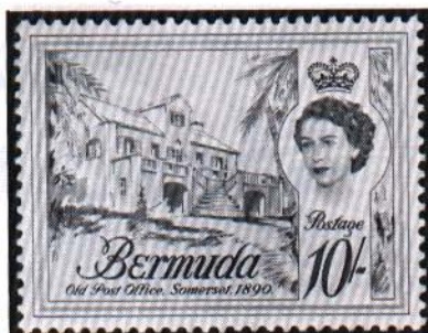
Fig. 10. Somerset Post Office, 1890 [Sc. 190, 1962]
